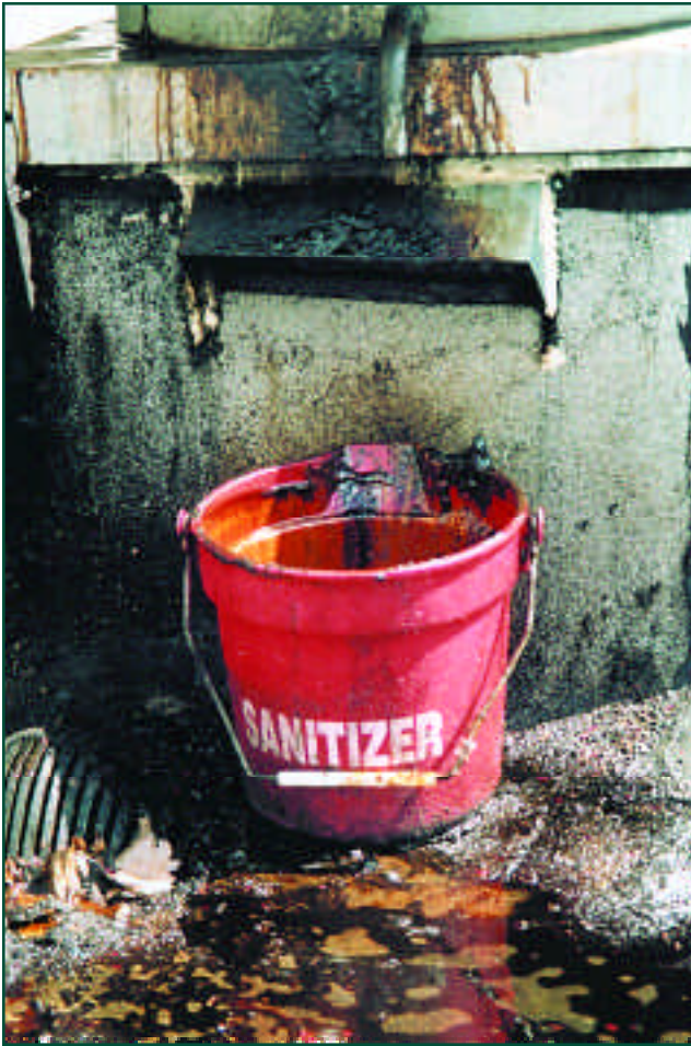
Photo 2: Rooftop grease spilling into a roof drain is stormwater pollution.
